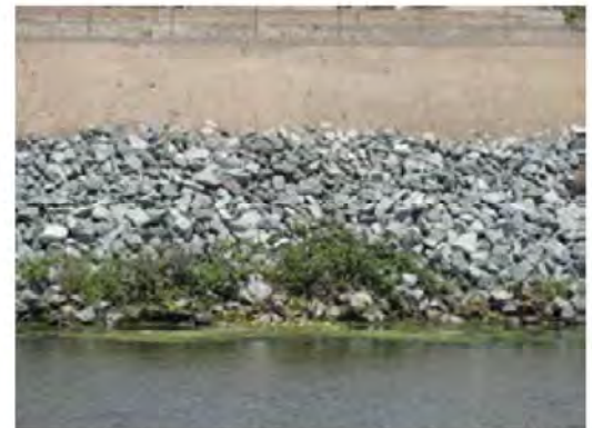
Close view of the repaired site.
