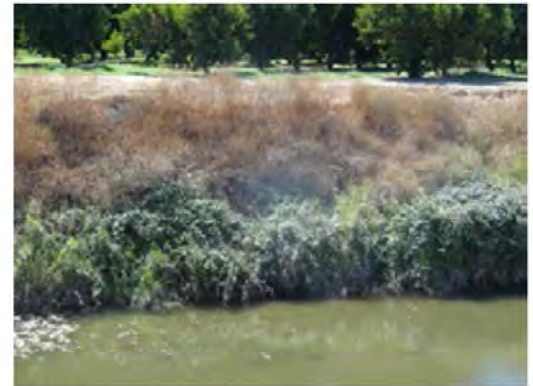
Front view of repaired site.
