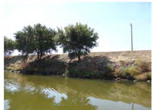
View of the site from downstream.
