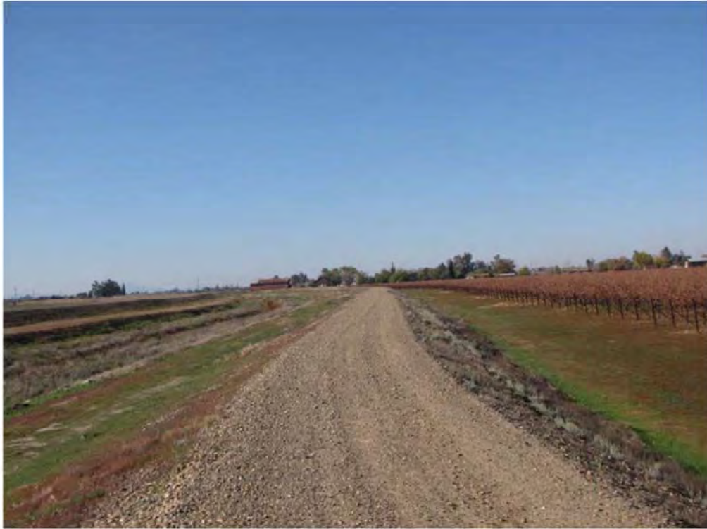
Acceptable Vegetation Maintenance: Good grass coverage with no grass or brush over 12" tall
