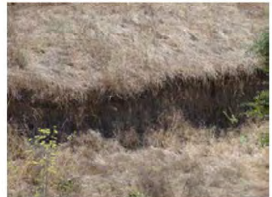
Closer view of the erosion.
