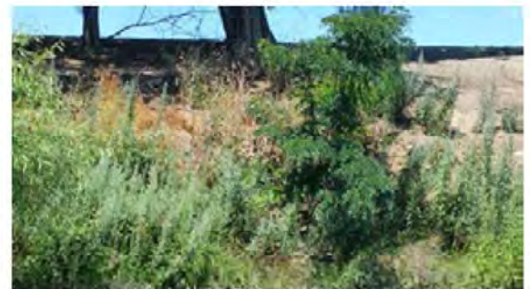
Close view of the site. Note large trees at the levee shoulder.
