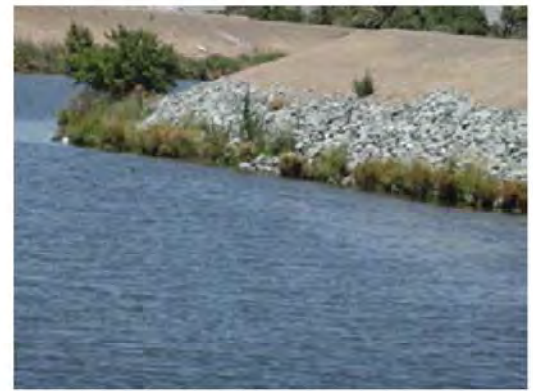
Front view of the repaired site.
