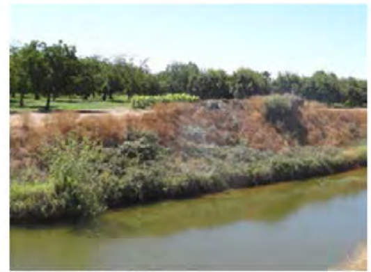
View of the repaired site.
