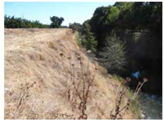
Downstream view of the site.
