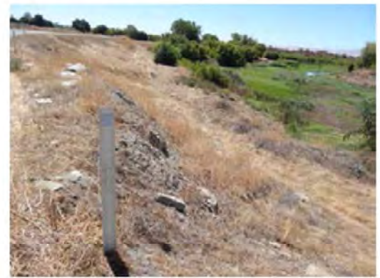
Looking upstream at the site.
