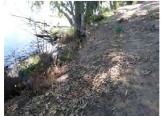
Front view of the erosion. Dense vegetation is visible.
