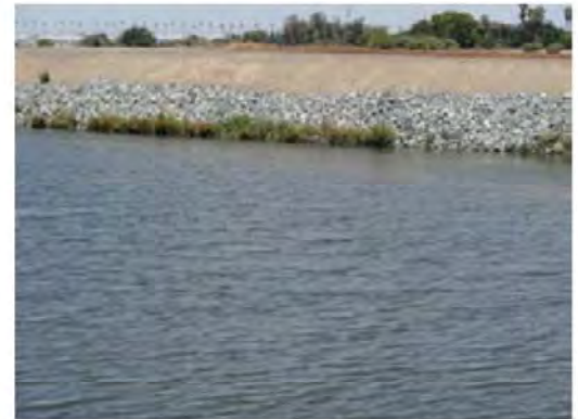
Front view of the of the repaired erosion site.
