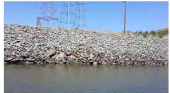
Front view of the repaired site.
