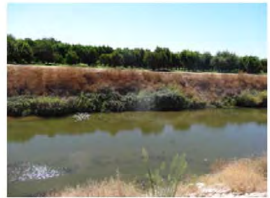
Front view of repaired site.
