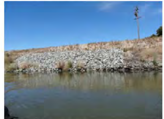
Front view of the repaired site.
