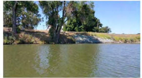
Upstream view of the repaired site.
