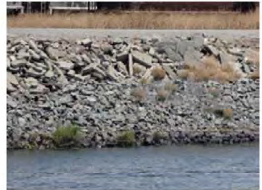
Close view of the repaired erosion site.
