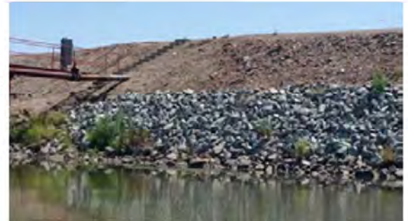
Close view of the repaired site.
