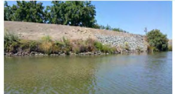
Front view of the repaired site.
