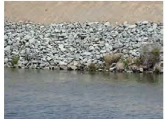
Front view of the repaired erosion site.
