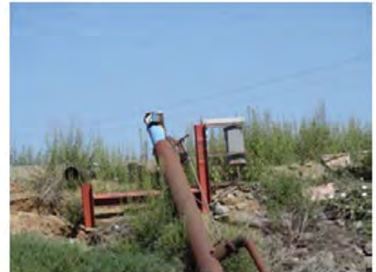
Close view of the erosion. Vegetation around the site is visible.
