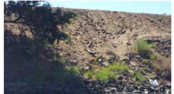
Front view of the repaired erosion site.
