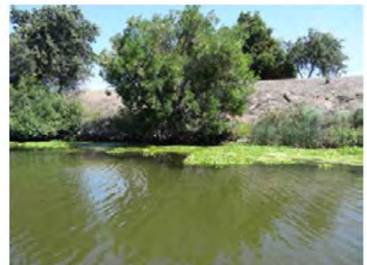
Front view of the erosion.
