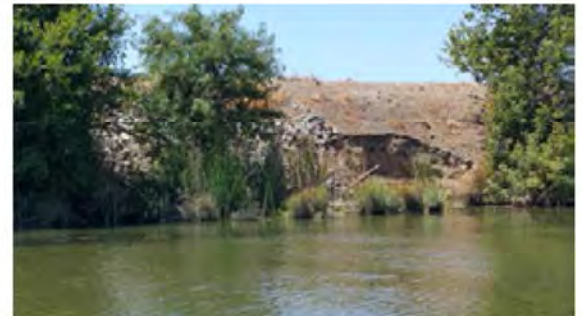
A close view of the erosion.
