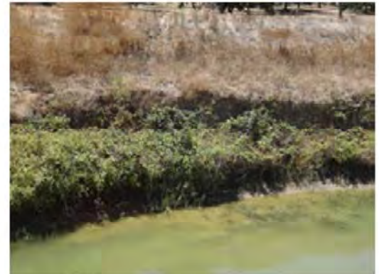
Closer view of the erosion.
