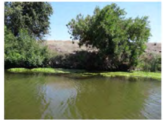
View of the erosion from the survey boat.
