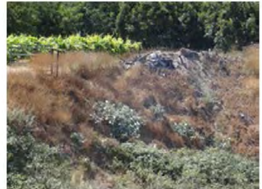
Front view of the repaired erosion.
