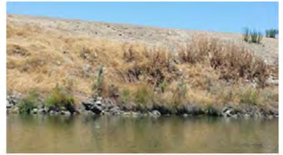
Direct view of the site.
