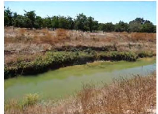
Close view of the erosion.
