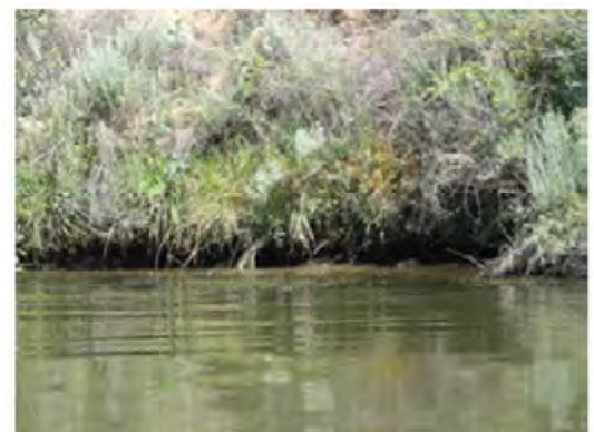
Front view of the site. Note the erosion is invisible because of the dense vegetation.
