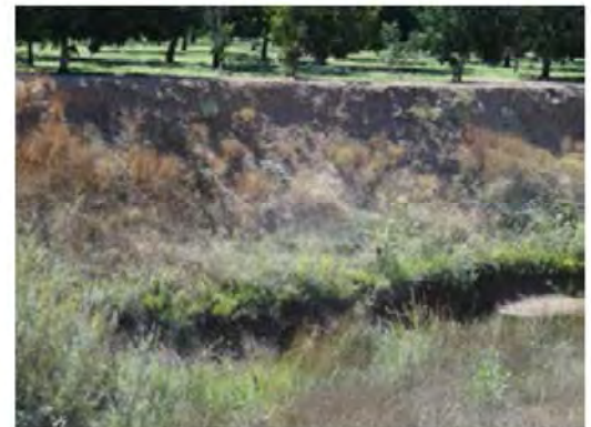
A close view of the erosion.
