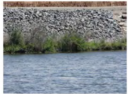
Front view of the repaired erosion site.
