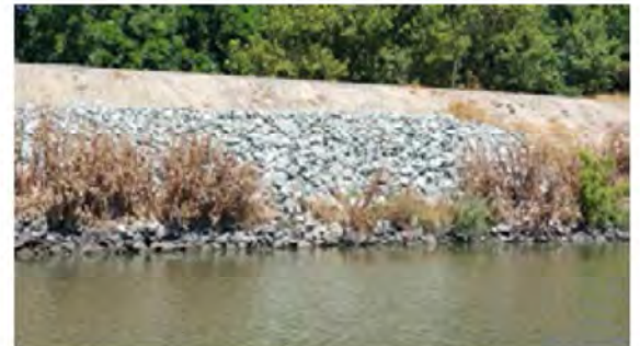
View of the repaired site.
