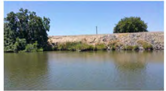
Direct view of the site.
