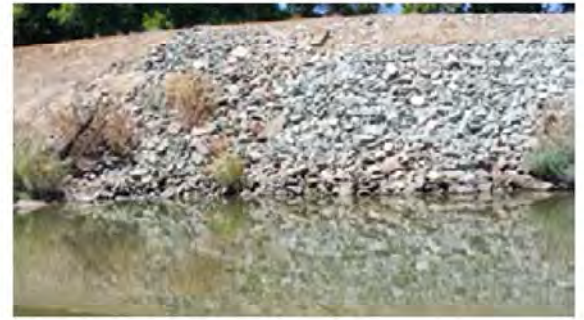
Upstream view of the repaired site.
