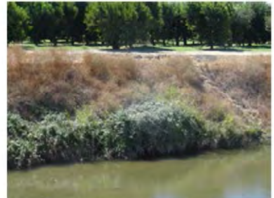
A closer view of the repaired site.
