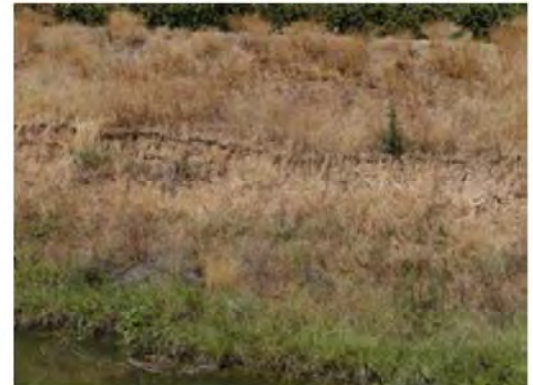
Close view of the erosion.
