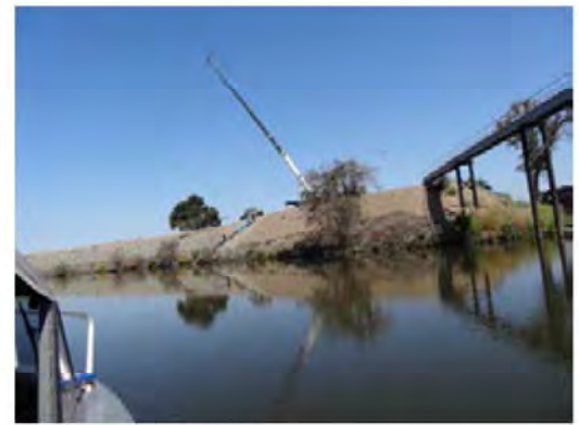
Front view of the erosion.
