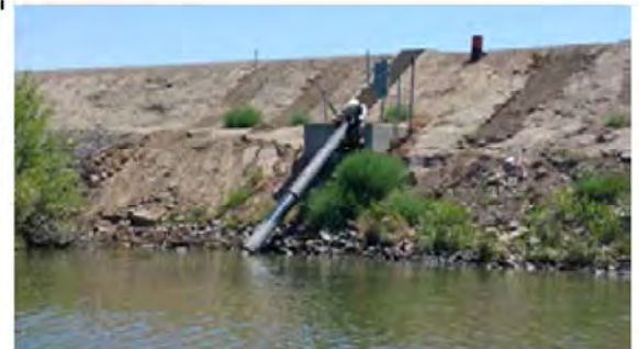
Close view of the repaired erosion site.
