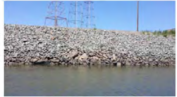
Front view of the repaired site.
