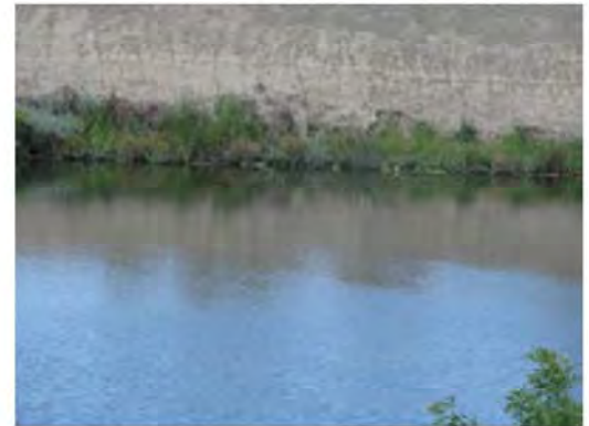
Front view of the erosion.
