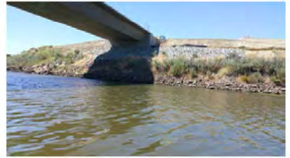
Front view of the repaired site.
