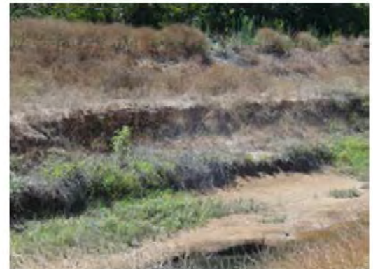
Close view of the erosion.
