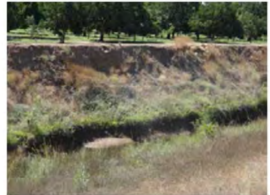
Close view of the erosion.
