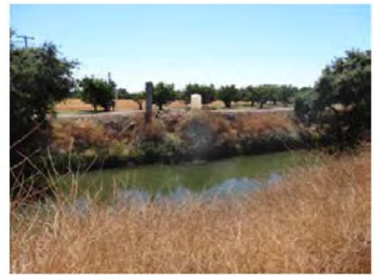
View of the erosion site.
