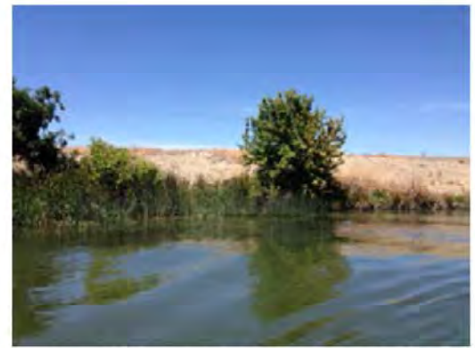
Front view of the erosion. The tree and vegetation block the view of the site.
