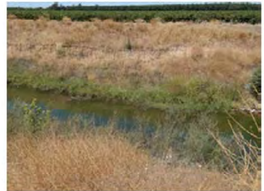
Close view of the erosion.
