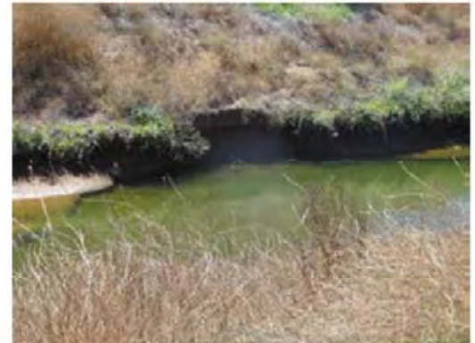
Close view of the erosion.
