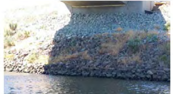
Front view of the rip rap.
