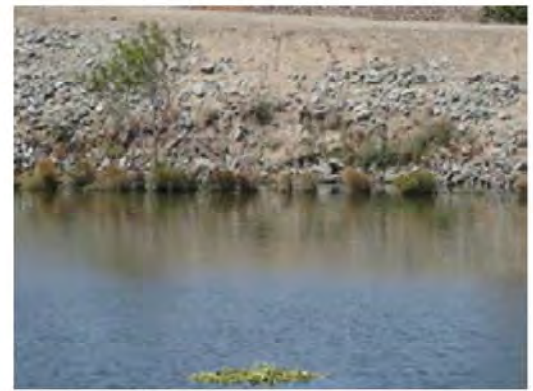
Front view of the erosion.
