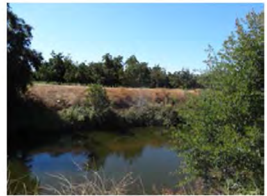
Front view of the erosion site from the left river bank.
