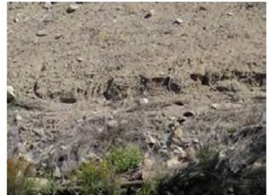
Close view of the erosion.
