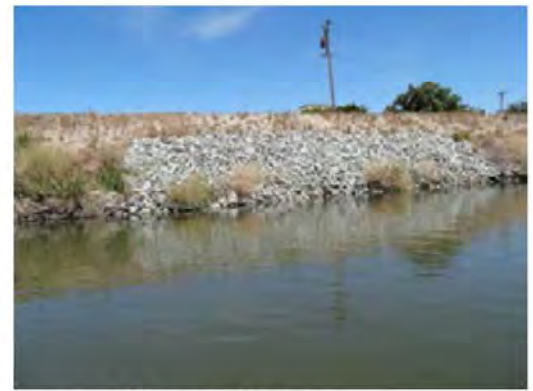
Front view of the repaired site.
