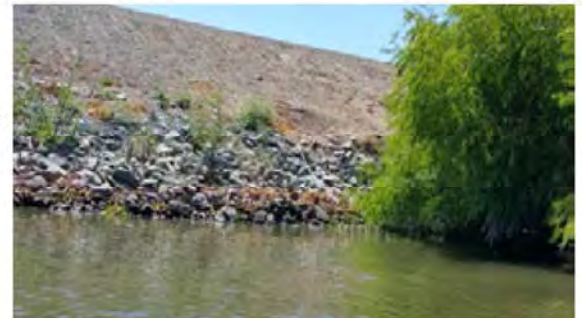
Close view of the repaired erosion site.
