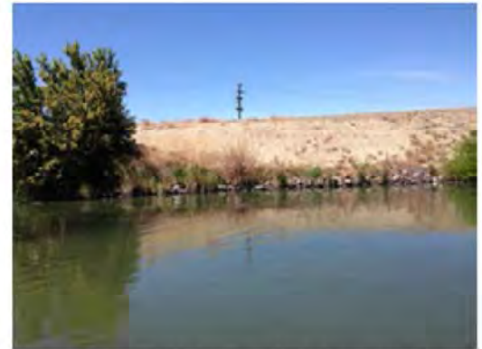
The erosion is invisible because of the dense vegetation.
