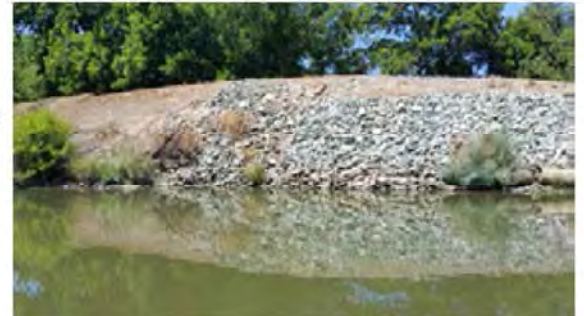
Close view of the repaired site.
