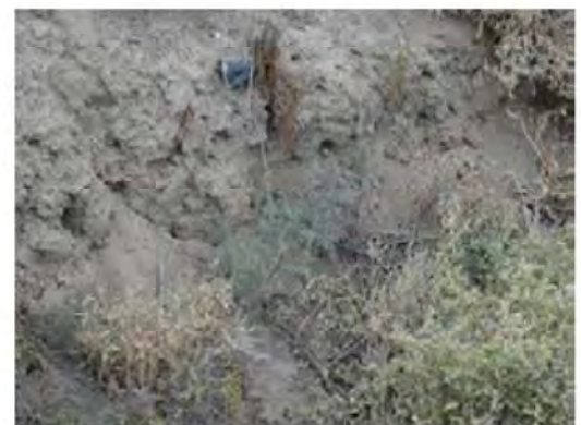
Close view of the erosion.
