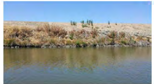
Close view of the erosion.
