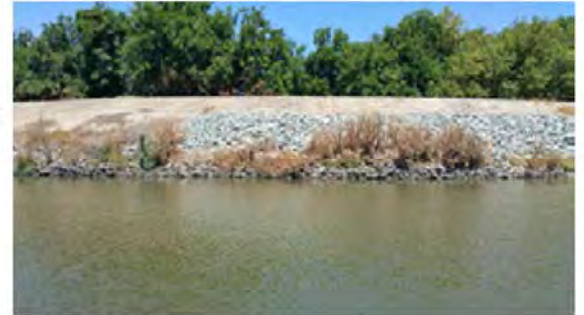
View of the repaired site.
