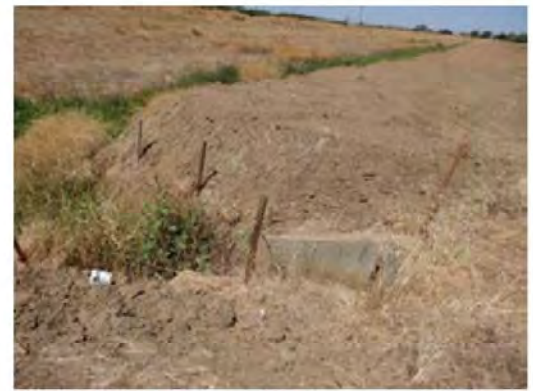
Looking at the repaired erosion site.
