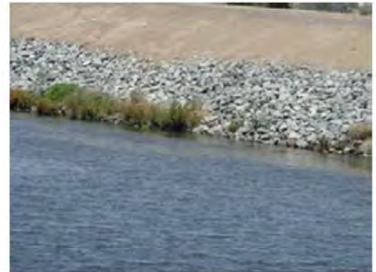
Front view of the repaired site.
