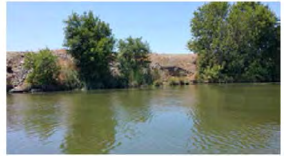
Front view of the erosion. Note the riprap protection near the site.
