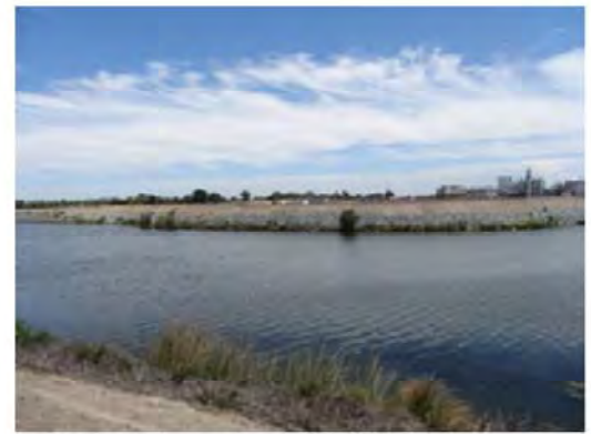
Front view of the repaired erosion site.
