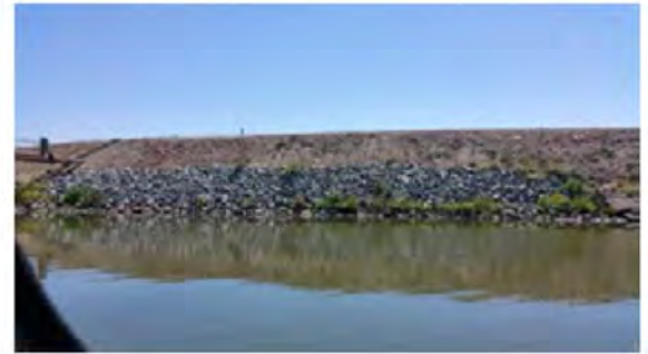
Front view of the repaired site.
