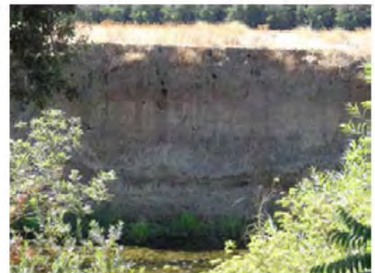
Close view of the erosion.
