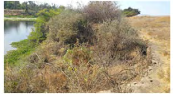
Close view of the erosion.
