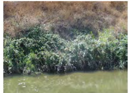
Close view of the repaired site.
