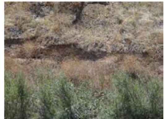
Close view of the erosion.
