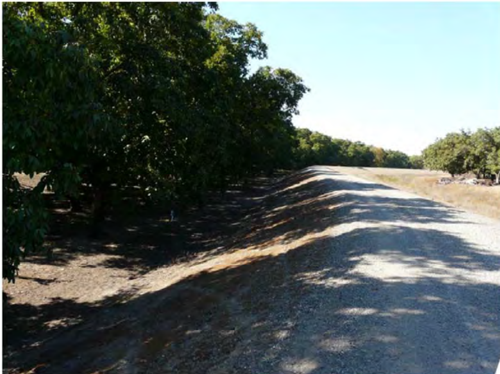
Acceptable Tree Maintenance: No limbs within 5' of the levee obstruct visibility or access
