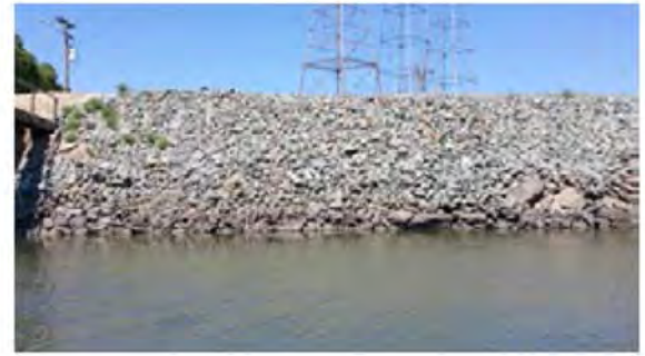
Front view of the repaired site.
