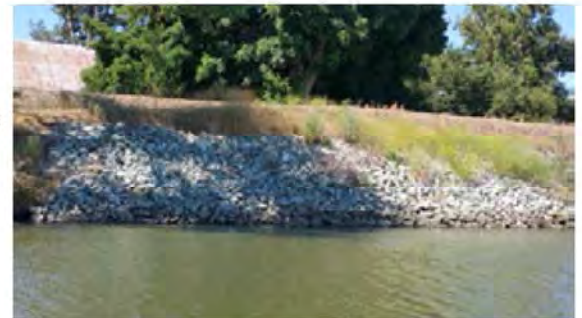
Front view of the repaired site.
