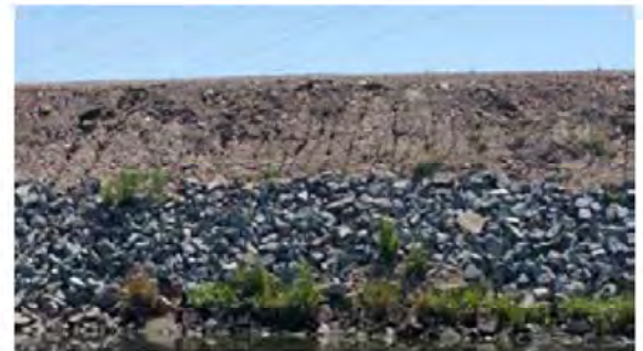
Close view of the repaired site.
