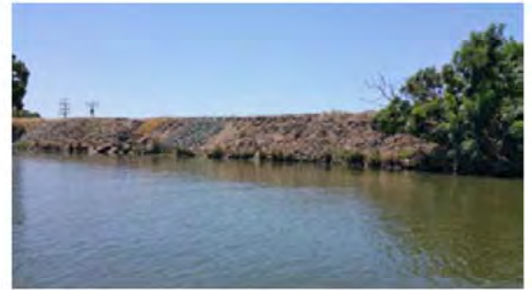
Downstream view of the site.
