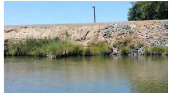
Direct view of the site.
