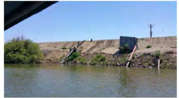
View of the repaired erosion site from the survey boat.
