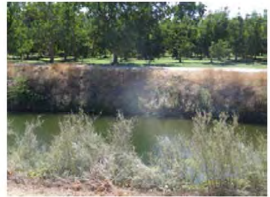
Front view of the erosion.
