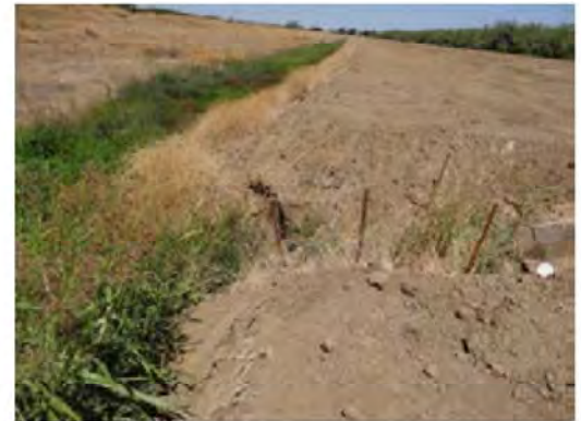
The erosion site has been repaired and vegetation has been removed.
