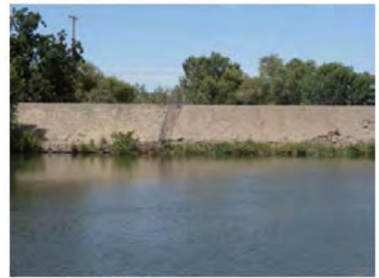
Front view of the erosion site.
