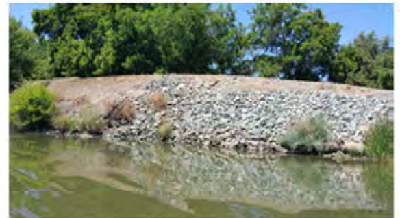
Closer view of the repaired site.
