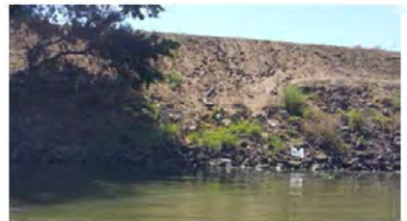
Close view of the repaired erosion site.
