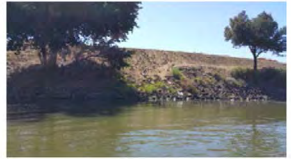
Front view of the repaired site.
